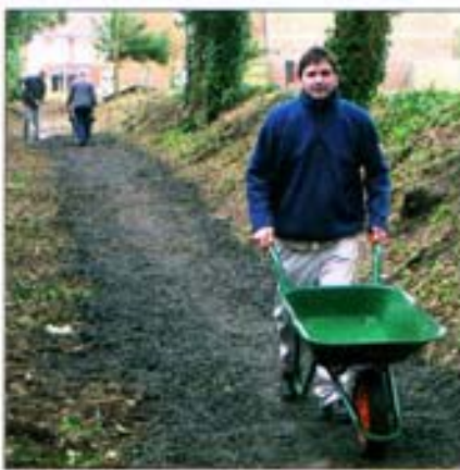
Young offenders at work on the Edenham Project
